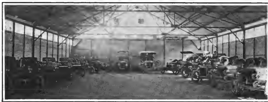
GARAGE BUILT OF ANGLE IRON, CORRUGATED IRON AND CONCRETE, RECENTLY OPENED IN HONOLULU, HAWAIIAN ISLANDS.
